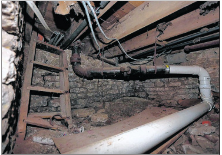
A once-hidden basement crawl space, one of two in the house, is thought to have been a hiding place for escaped slaves.
